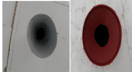
Figure 3: Typical floor diffusers
